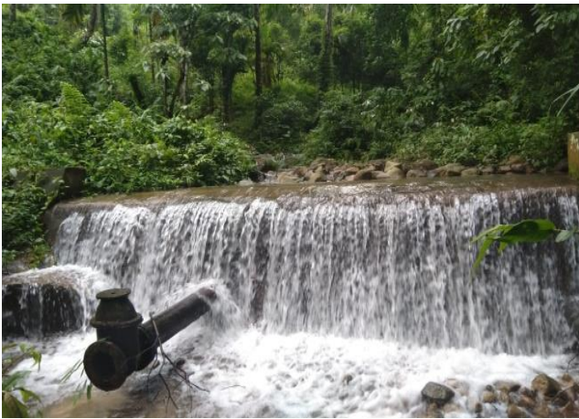
Fig. 1. Construction of dam at source for water supply at Warisep Stream at the foot of Tura Peak.
